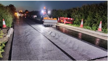
**Station Road Reconstruction** involved upgrading and re-surfacing of 1,485m of the existing country lane linking the A41 with Quainton village as far as the location of the HS2 site access, in order to accommodate the unrestricted two-way movement of vehicles and HGV's servicing HS2 construction works.
