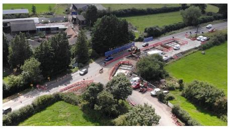
The Project required the complete reconstruction of 1.5 km of the existing Station Road carriageway and also to complete improvements to the existing priority junction of the A41 and Station Road, in order to cater for the increased traffic flows associated with HS2 construction work. The A41 carries traffic from Bicester to Aylesbury and Station Road serves the village of Quainton, with the access to the HS2 works site compound circa 1700m along Station Road.
